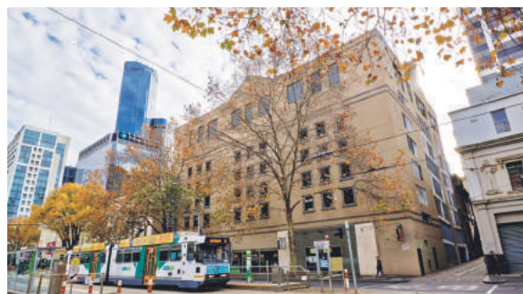
The Group invested in Australia with acquisitions of a commercial building and two data centres
