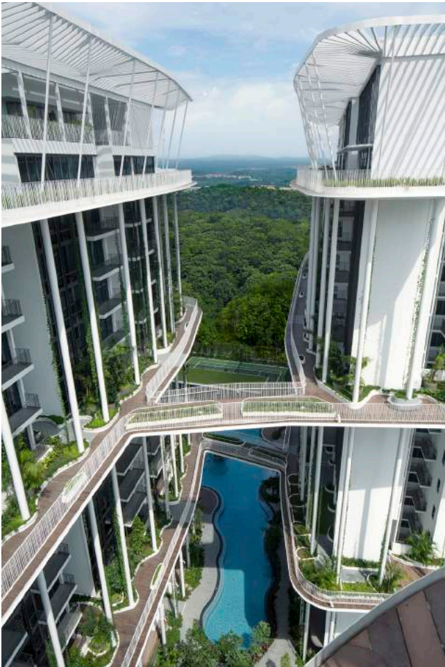
^ Sky links on the 6 th and 12 th storeys of The Tembusu connect all five blocks of the freehold development at the Group's former headquarter site
