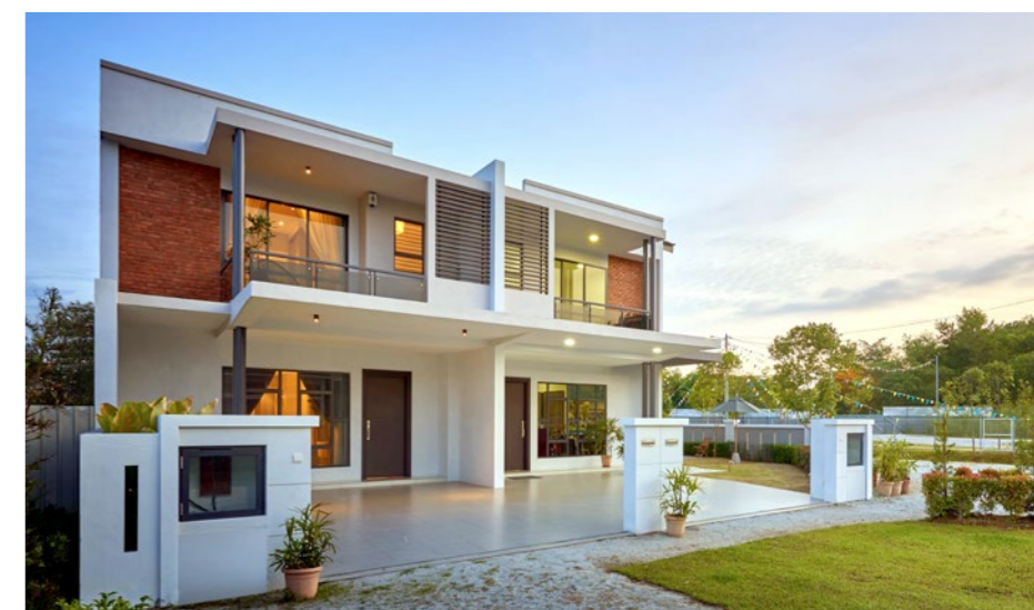
Garden Superlink in Penang comprises 145 units of double-storey terrace houses offering extended features for the whole family, including generous green spaces for gardening.
