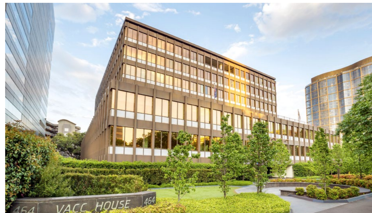
464 St Kilda Road is a freehold 8-storey office building with striking views over Albert Park Lake in Melbourne, Australia.
